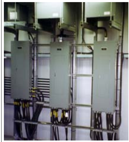
Figure 2-2 Electrical distribution panel
