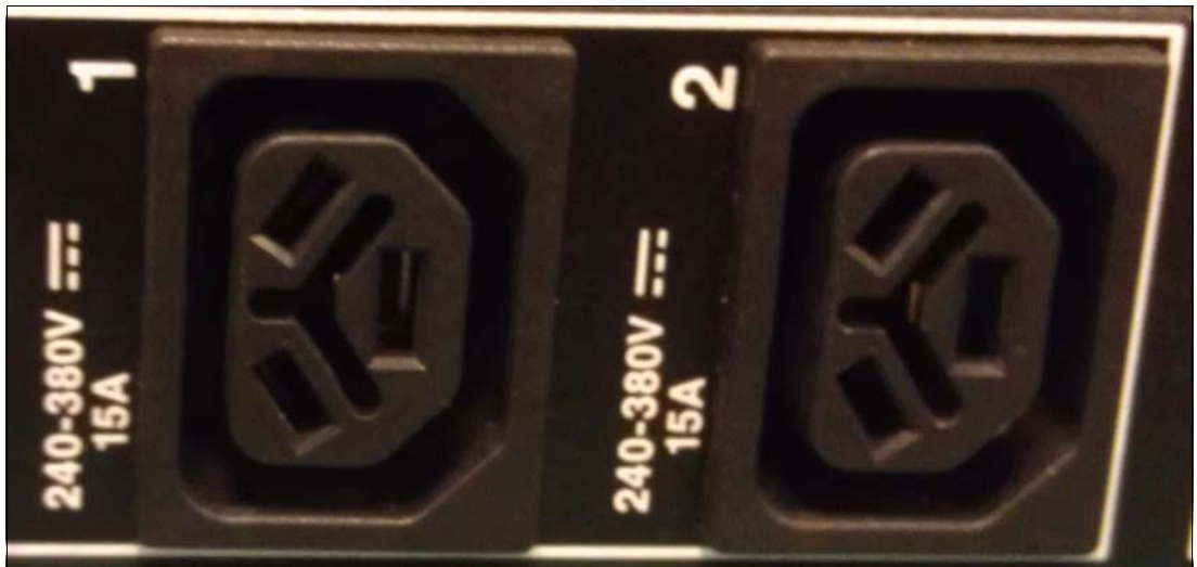
Figure 4-10 HVDC PDU RF-203P outlets
