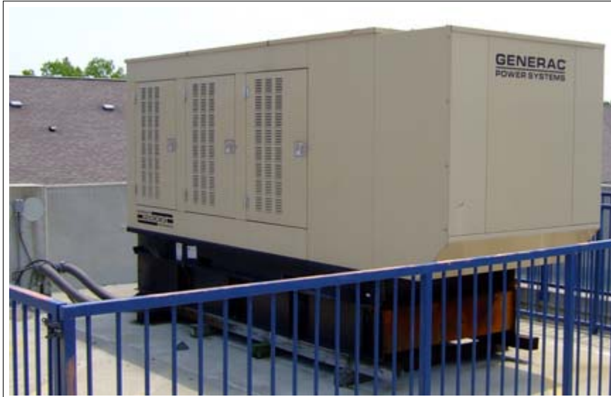
Figure 2-6 External generator on top of a building
