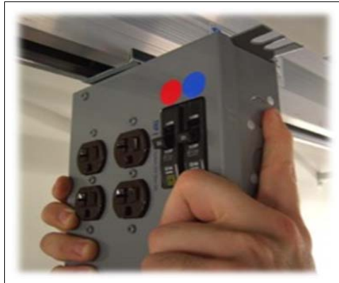
Figure 2-10 Tap-off box with power outlets
