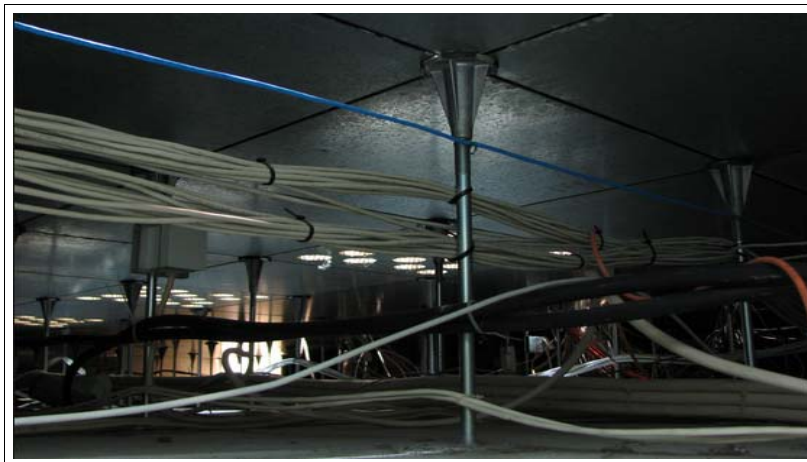
Figure 2-8 Power whips and networking cables under the raised floor in a data center
