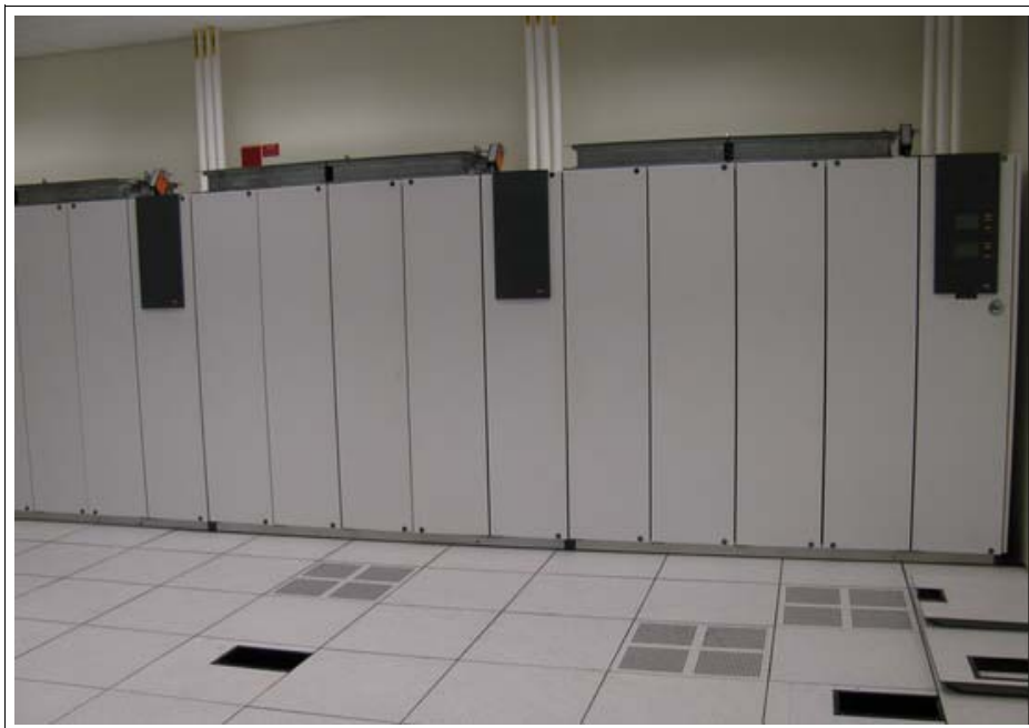
Figure 2-19 Computer room air conditioner
