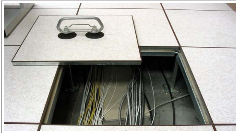
Figure 2-7 Raised flooring with networking and power cable whips
