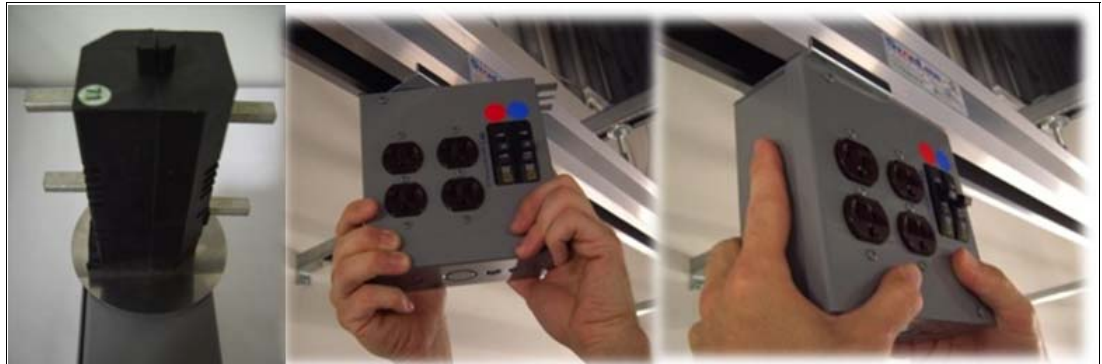
Figure 2-9 Tap-off box twist locking into busway
