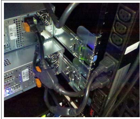
Figure 2-16 Server to PDU line cord connection
