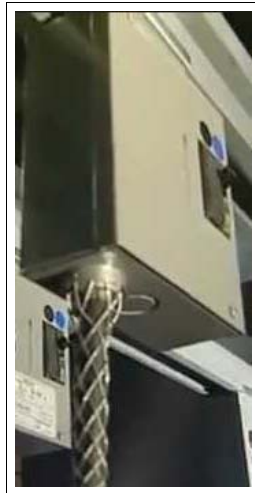
Figure 2-11 Tap-off box with main power cable whip
